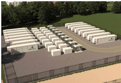
The United Kingdom's first grid-scale battery 2 MW
