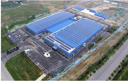
World's largest VRFB project in Dalian, China 800 MWh/200 MW
